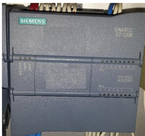
Figura 2: PLC S7-1200 CPU 1212C AC/DC/RLY, ONBOARD I/O.
