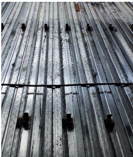
Gráfico 51: Headed Studs in Steel Deck System.
