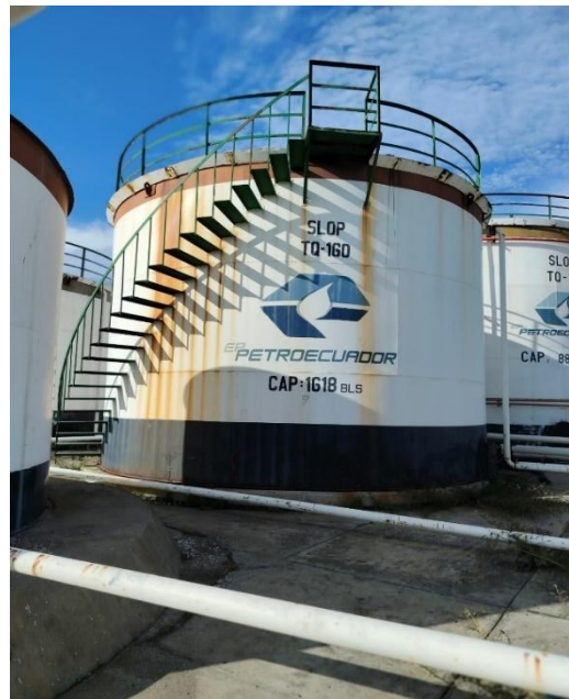
Figura 8: Tanque de Slop #160
