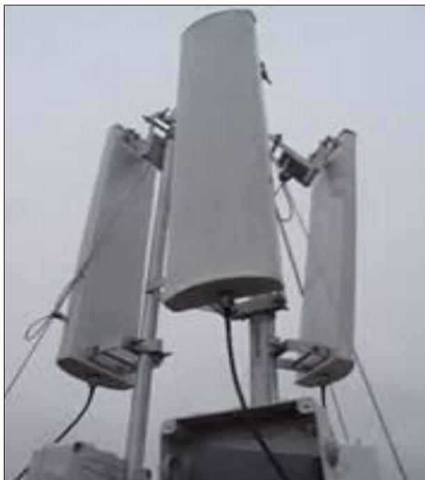
Figura 21: Antena sectorial: Cisco
