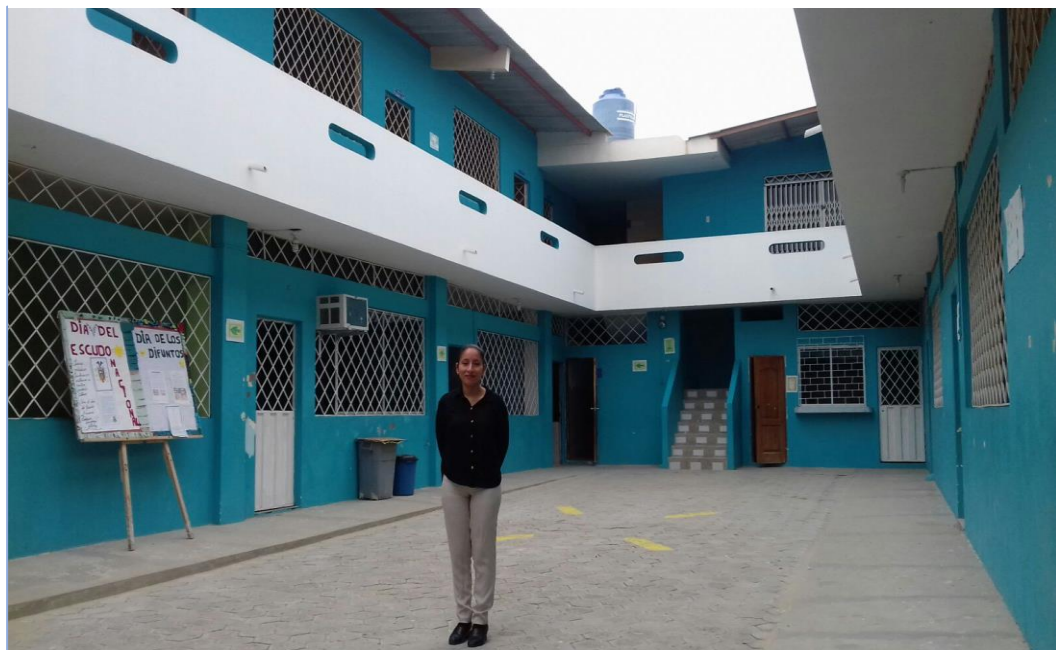
Classrooms At Colegio "Prof. Ernesto González Muñoz".
