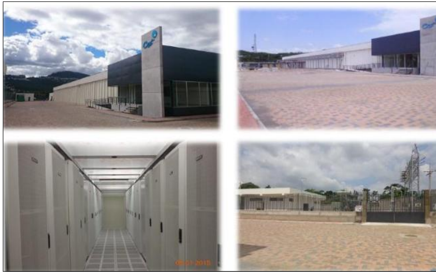
Figura 10. Data Center Cnt Cloud, (CNT Cloud, 2016).
